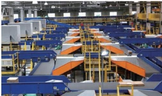
Shenzhen Air Mail Processing Center Site
