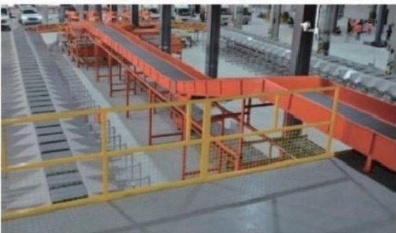
Hangzhou Yuantong Secondary Warehouse Site Photo 2
